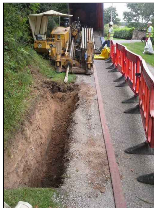
Typical Drilling Rig/Launch Pit
